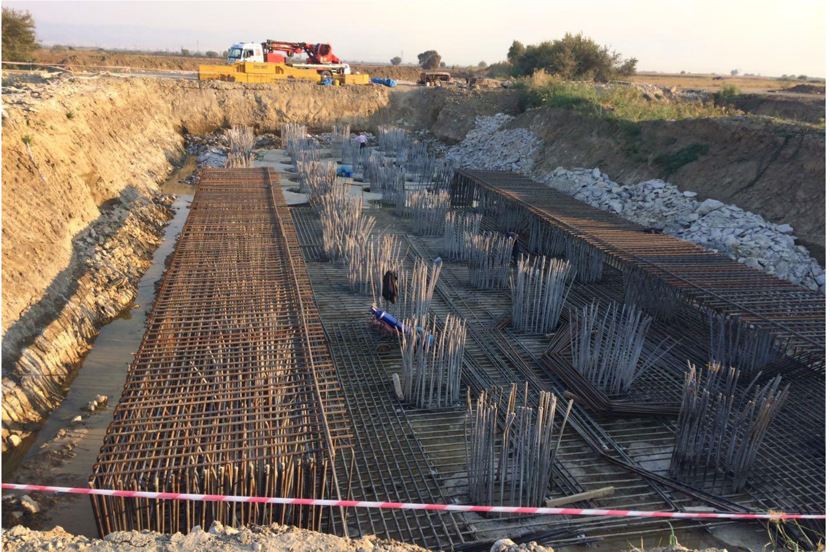
Foundation Iron - Pile Anchors
