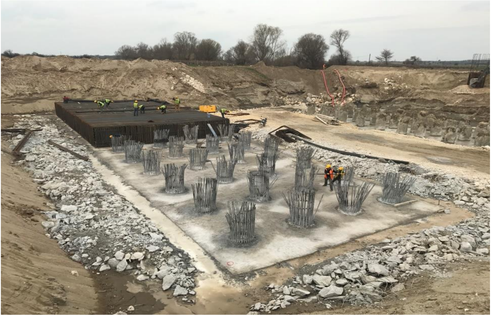
FOUNDATION IRON – steel piles
