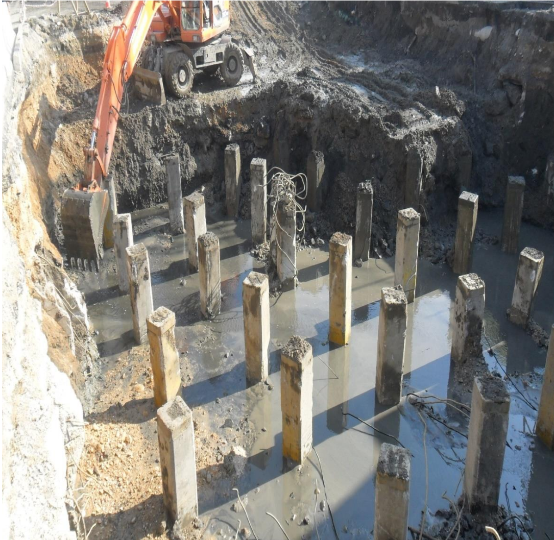
45*45 reinforced concrete piles
