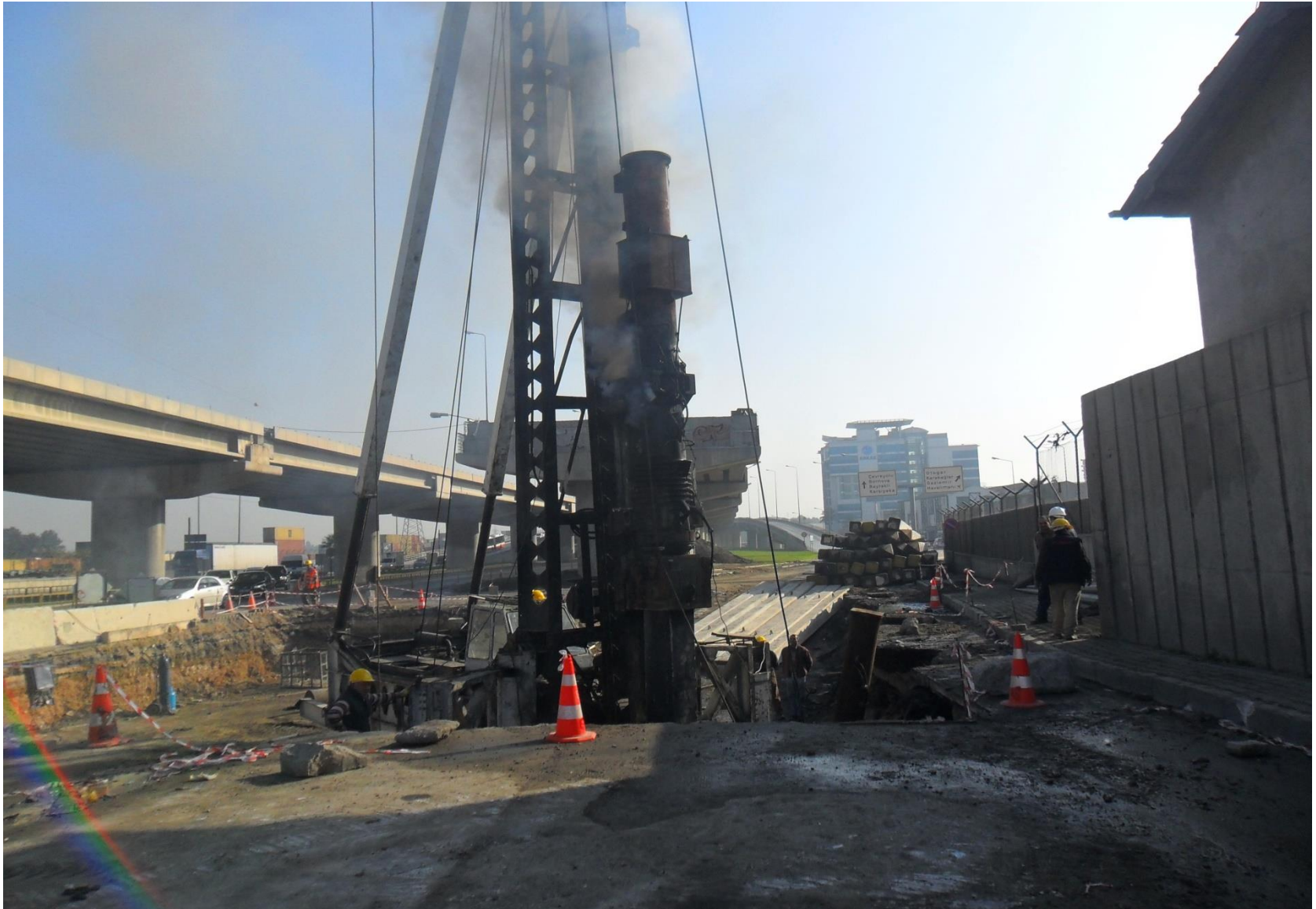
45*45 cm raker piles L=25-29 mt ( in two pieces )
