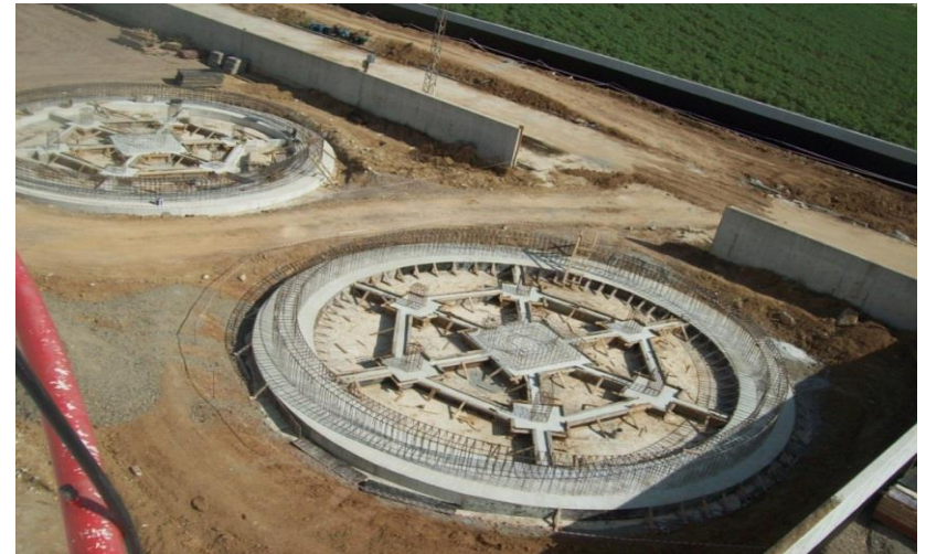
MARMARA WAREHOUSING TANK FOUNDATION
