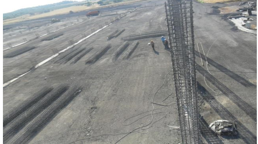
COLUMN IRON AND MOLD PREPARATIONS
