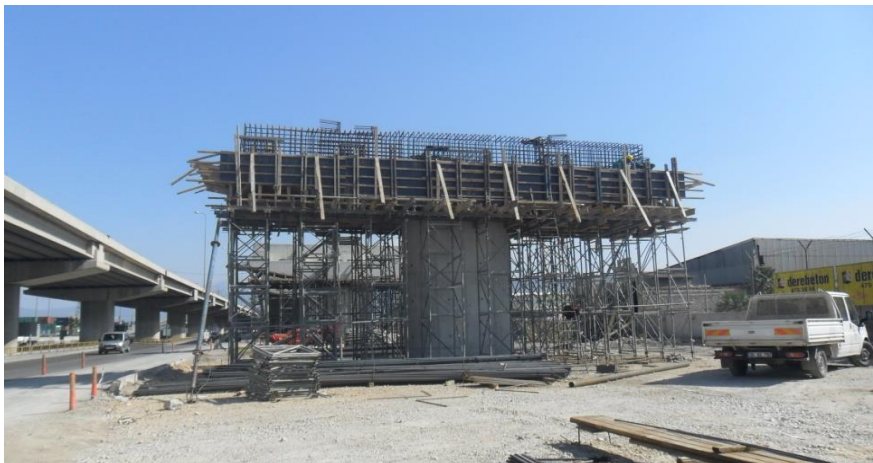
FOUNDATIN – HEAD BEAM WORKS
